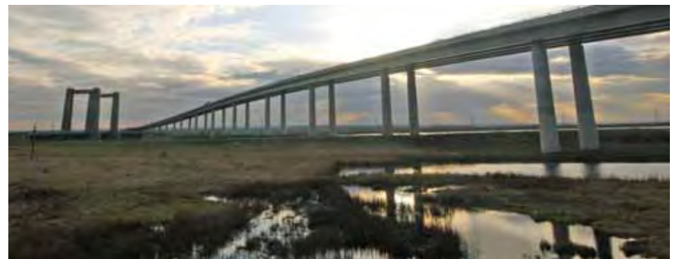
Sheppey Bridge, North Kent
