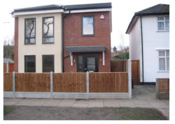
**Features:** Solar Thermal Panels, which are estimated to contribute 18% of the annual energy needs for the tenants. Built to Code 4 standard. Lifetime homes and Secured by Design achieved. DDA Compliant, fully adaptable with provision for hoist, through floor lift and/or stair lift.
