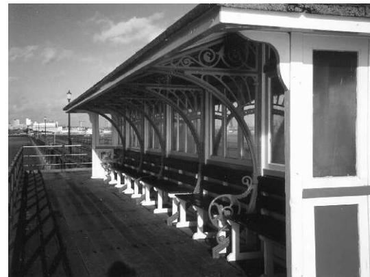
The present Pier dates from 1889
