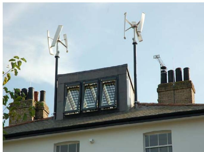
Chalkwell Hall in Chalkwell park has been fitted with a variety of renewable energy technologies including micro wind turbines, solar PVs & solar thermal panels and a biomass boiler system.
