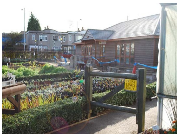
This building at the 'Growing Together Community Garden' is constructed of straw bales which have then been clad with timber boarding.
