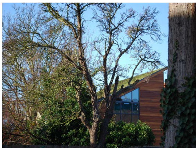
A green roof on a new development in Milton.
