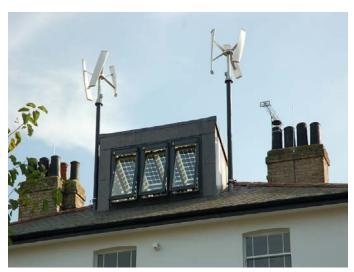
Chalkwell Hall in Chalkwell park has been fitted with a variety of renewable energy technologies including micro wind turbines, solar PVs & solar themal panels and a biomass boiler system.
