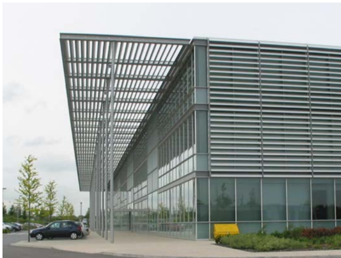
Bris Soleil sun shading on the south elevation of the Royal Bank of Scotland offices in Prince Avenue.
